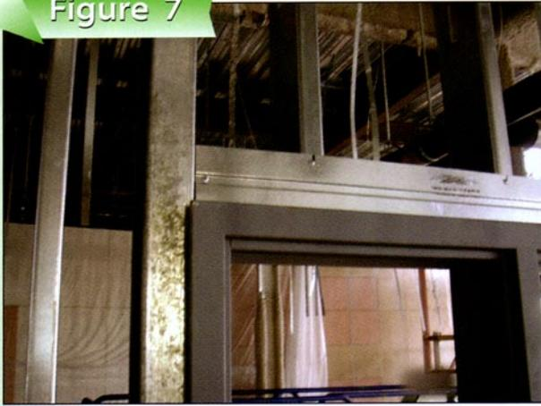
*The screws that connect the header to the vertical king stud are placed in recessed channels that are roll-formed into the product. The finished surface is then aligned with adjacent studs so there is no overlap of material.*
