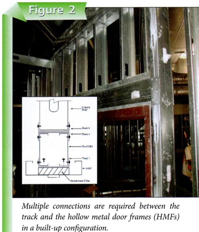
*Multiple connections are required between the track and the hollow metal door frames (HMFs) in a built-up configuration.*
