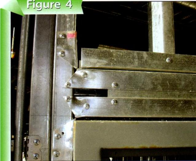
*Studs and tracks are commonly hand-cut to size. They are dog-eared on each end, fastened with multiple screws, and often welded, depending on the skill and preference of the installer.*
